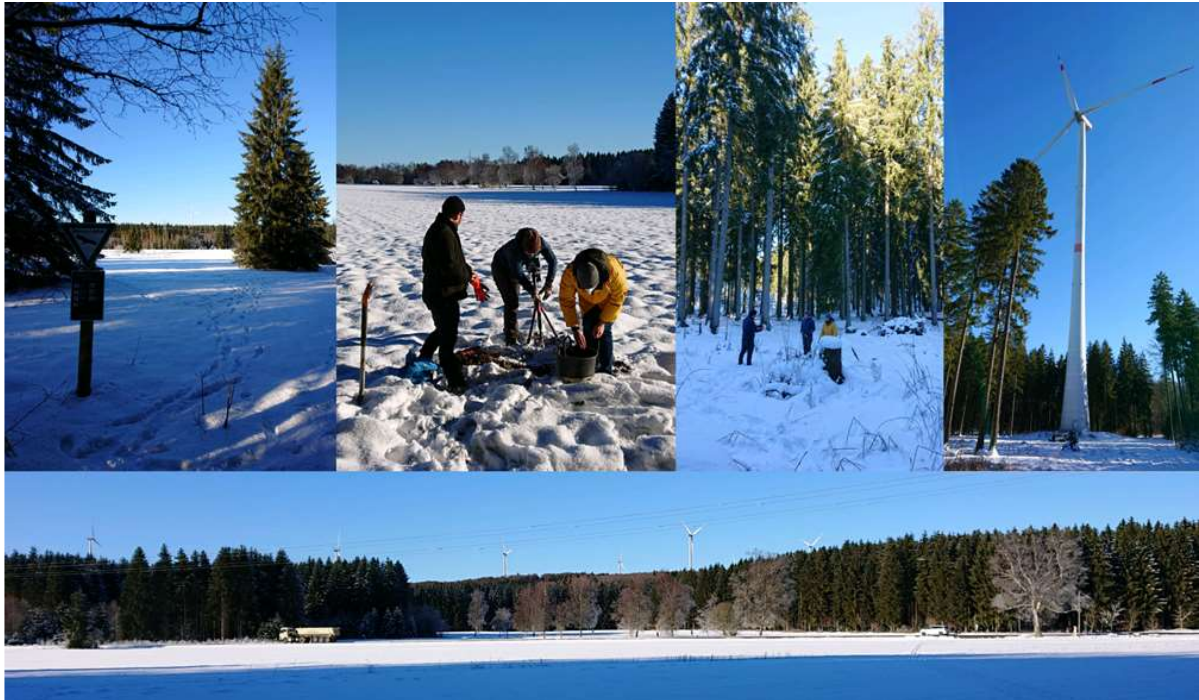
Figure 2: Impressions from the installation of instruments at wind farm Lauterstein in January 2022 for a measurement line of 5 km length oriented towards the east of the WTs. One instrument was installed on the foundation of a WT, the other instruments on fields and forest ground. Photos: Laura Gaßner
